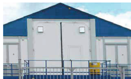
Indoor Distribution device ZRU-SESH 20/6 (6/20) kV
