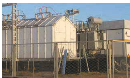
Indoor Distribution device ZRU-SESH of 35/6 kV
