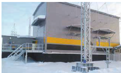
Indoor Distribution device with KRUE-110 kV
